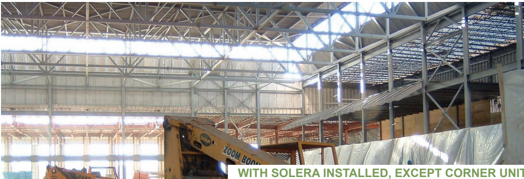
WITH SOLERA INSTALLED, EXCEPT CORNER UNIT
